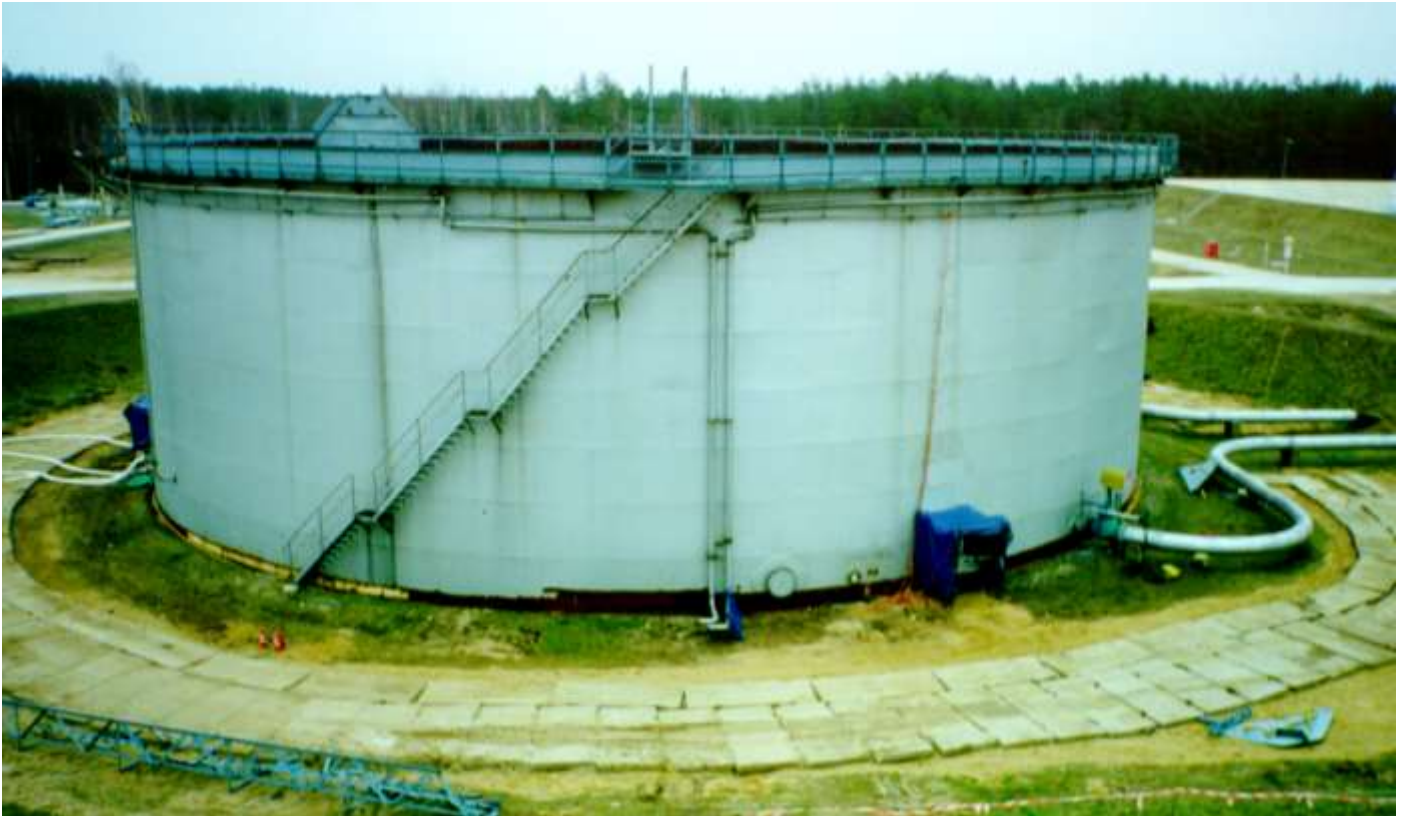
Fig. 2. General view of the tank
